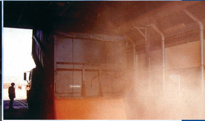
Above: Dumping prior to installing Burnley® Baffles.
